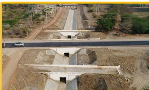
Main Canal completed stone lining
