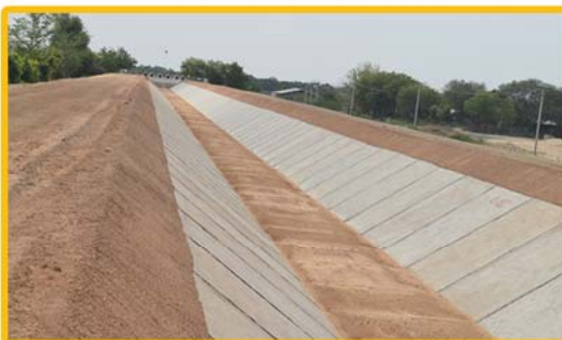
Left Main Canal completed concrete
