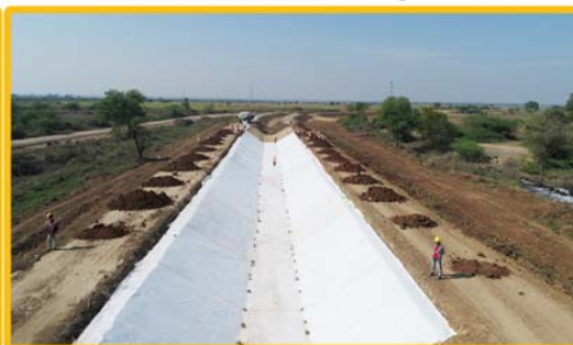
Right Main Canal geotextile laying
